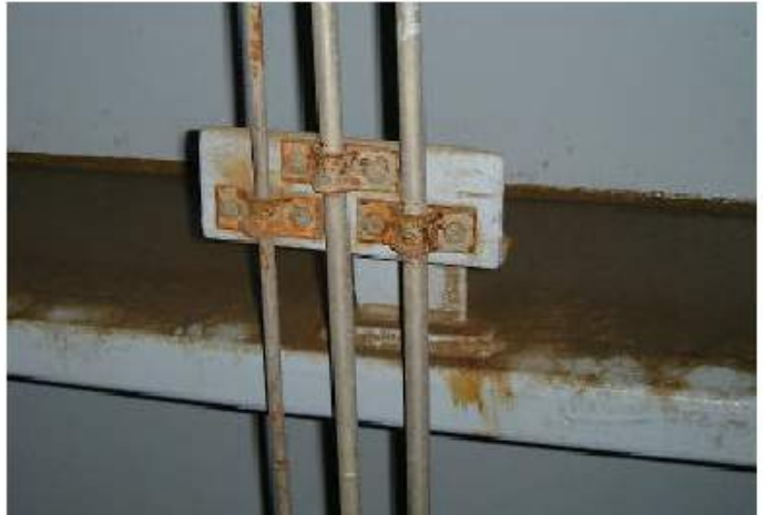
VRC tube in Ballast Tank 2
